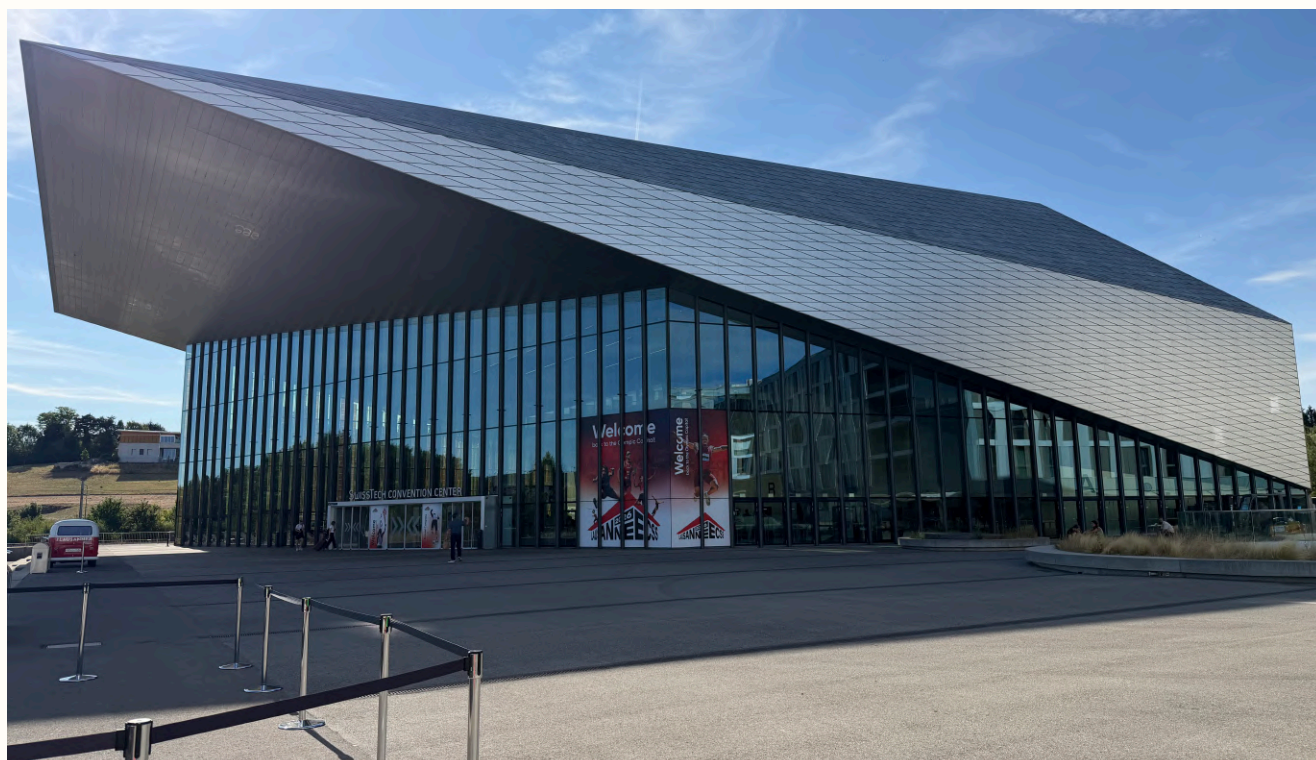
The SwissTech Convention Center at EPFL, dressed for ECSS Lausanne 2026 on the eve of the congress.
